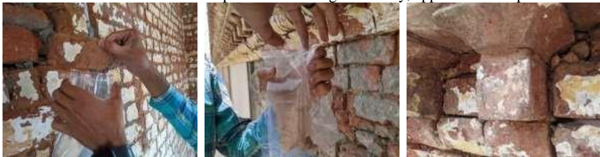
Figure 4. Sampling of deteriorated wall mortar for laboratory analysis
