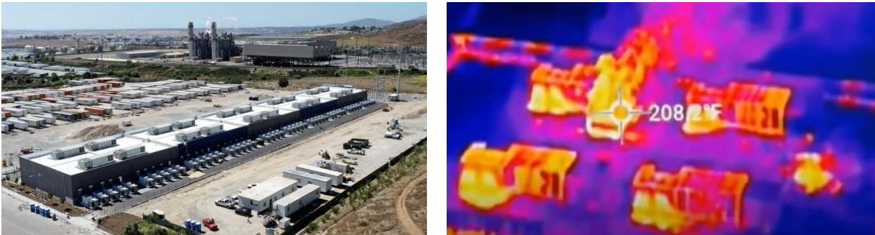
Fig. 2 Fire incident at the Gateway lithium-ion battery energy storage facility, USA
