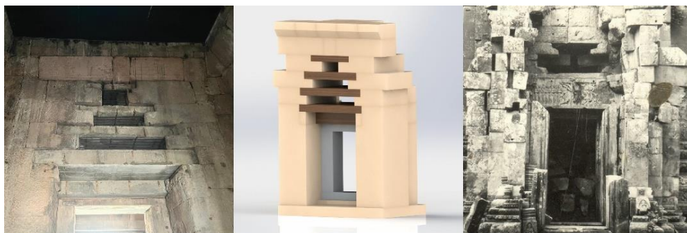
Figure 5 Demonstrates a wisdom technique to help receive and transfer weight over the door frame using the triangle principle. (Source: Kittisak Tammasakchai, 2025)
